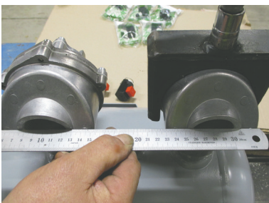
Check that all solenoid valves are in line with each other.
