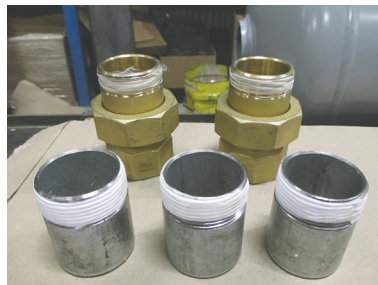
Pack all radiator unions and weld adapters with a suitable pipe sealant and screw them onto the air receiver.
